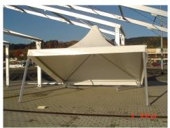
Lift one side of the structure and lock two legs in position, taking care not to trap the roof in the hinge, then bolt the flap closed.
