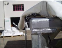
Slot each eave knuckle into the fabrication and bolt through holes and fit 4off round poles to eave so that they point to centre of tent. Then fit central spider with screw thread wound down.
