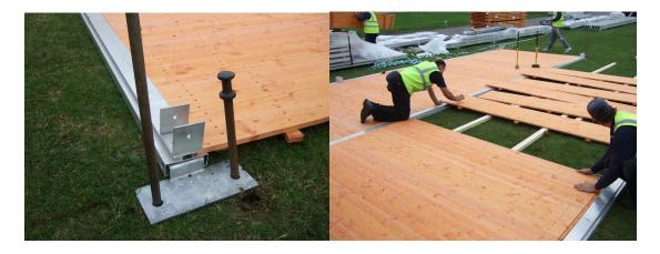
□ Repeat process until final bay then drive all stakes home. The marquee can now be laid out and installed as standard.
