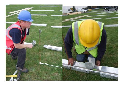
□ Attach gable-securing plate and lay rough-cut timber to chock floor. This will take up any bounce in floor allowing for unevenness in ground. It is recommended that 2 lines of 2"x 2" used in each bay at approx' 1/3 & 2/3 locations.
