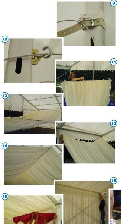
To stop the wire from pulling out or bowing when you attach the roof lining, attach a shackle 9 or lining clamp in the keder track **10** to every leg and secure the wire.
