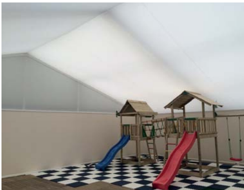
Tack-off Roof and Gables
